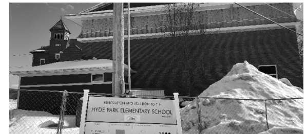
Hyde Park School District, 2017 Project
